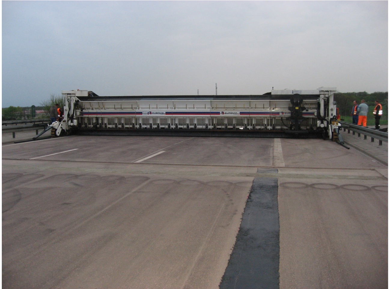
finisher KBR 110 SL with 14,5 m installation width, Eurovia Magdeburg construction side Vockerode
